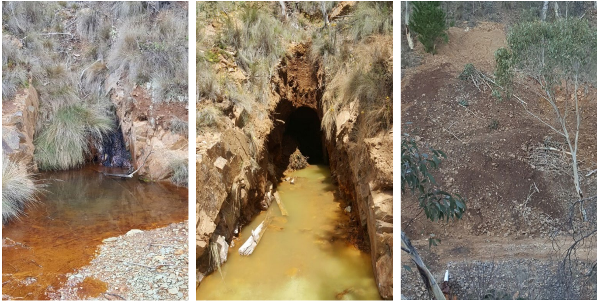
Fig. 1. Three images of the Nevada No. 1 Adit. From left to right, the images show the adit pre-, during and post-air entry control engineering works. Note the post-works adit drainage pipeline (white) at the bottom left of the image on the right.
