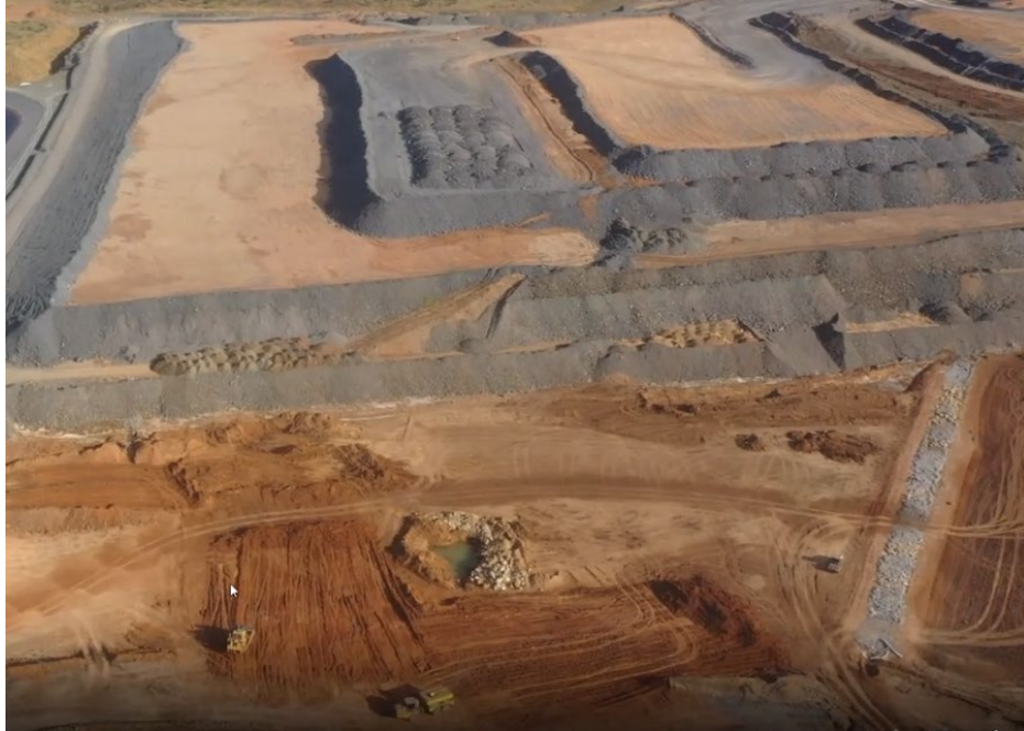
Fig 3. Paddock dumped PAF, outer NAF shell, and horizontal advection barriers (water trucks in foreground for scale)
