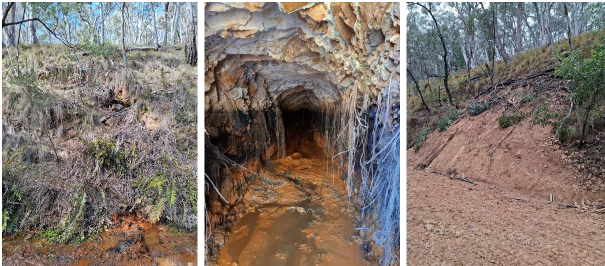
Fig. 2. Three images of the Nevada No.2 Adit. From left to right, the images show the adit pre-, during and post-air entry control engineering works. The post- second stage works adit drainage pipeline is buried beneath the road in the foreground of the image on the right.
