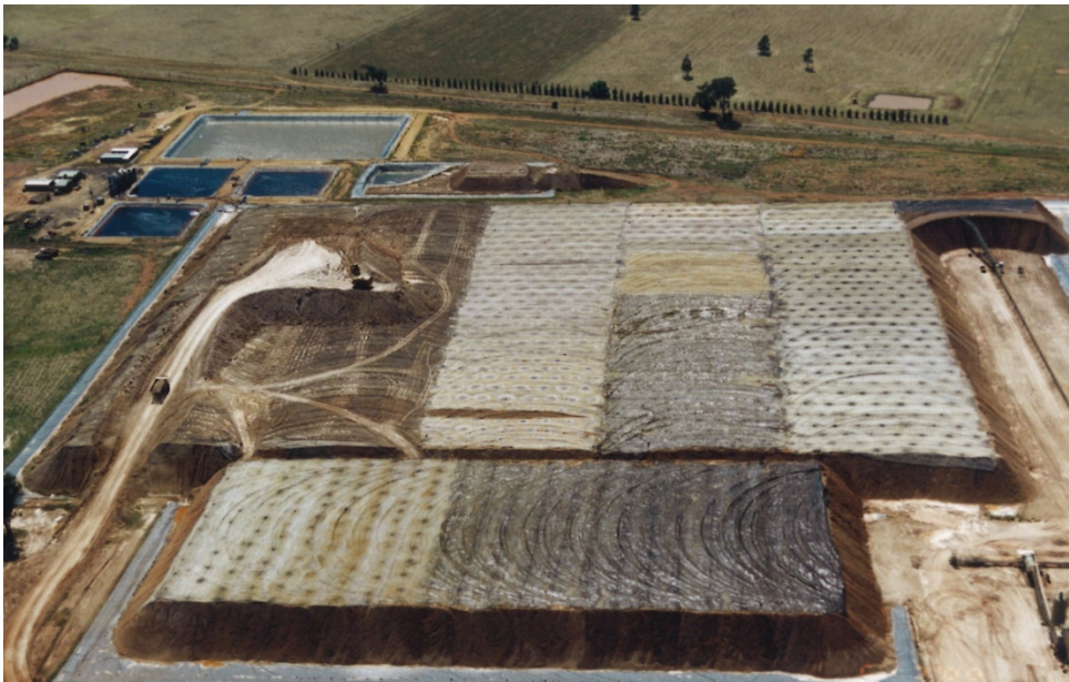
Figure 7: Dump leach construction on top of Heap Leach facility
