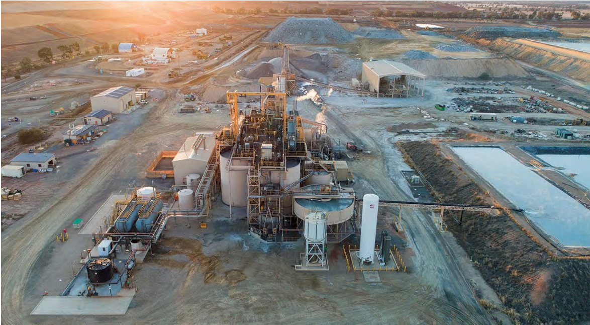
Figure 10: Tomingley Processing Plant (Source Alkane Resources)
