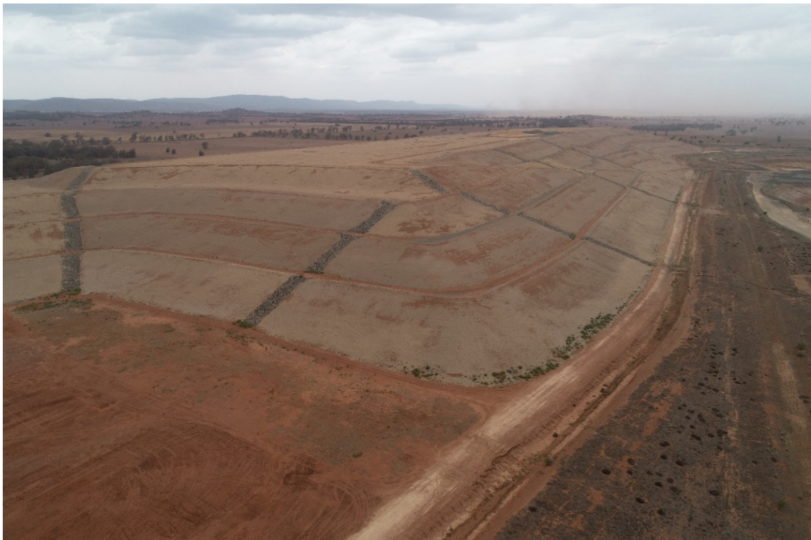
Figure 11: Rehabilitated Waste Rock emplacement-WRE3. (Source Alkane Resources)
