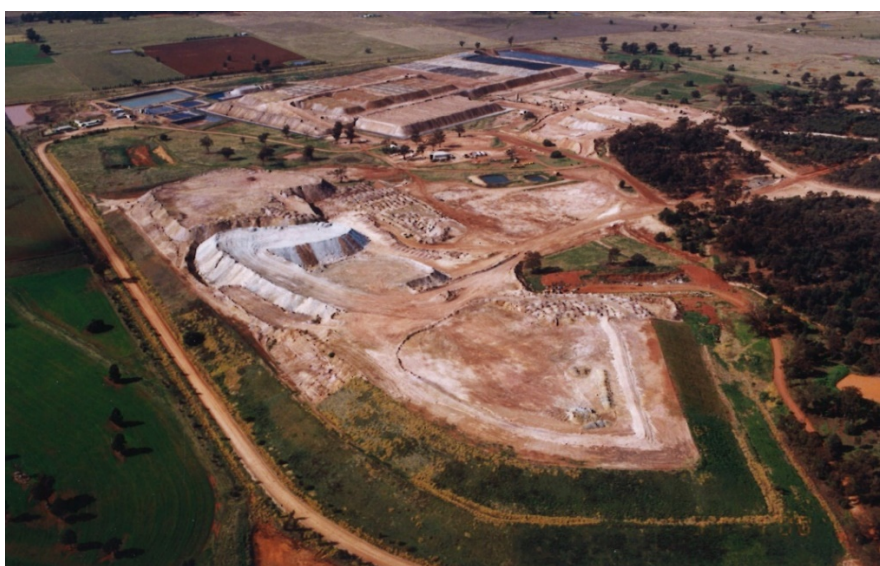
Figure 5: Peak Hill Waste Rock Emplacement under construction (Source Alkane Resources)
