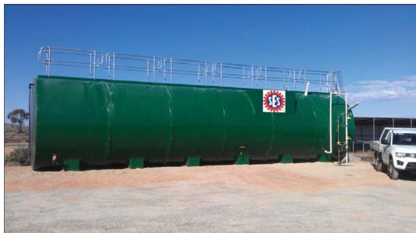
Fig. 4. SES Self contained 5 KL/hr ASS water treatment bio-reactor for building sites. Separate aeration plant not shown.
