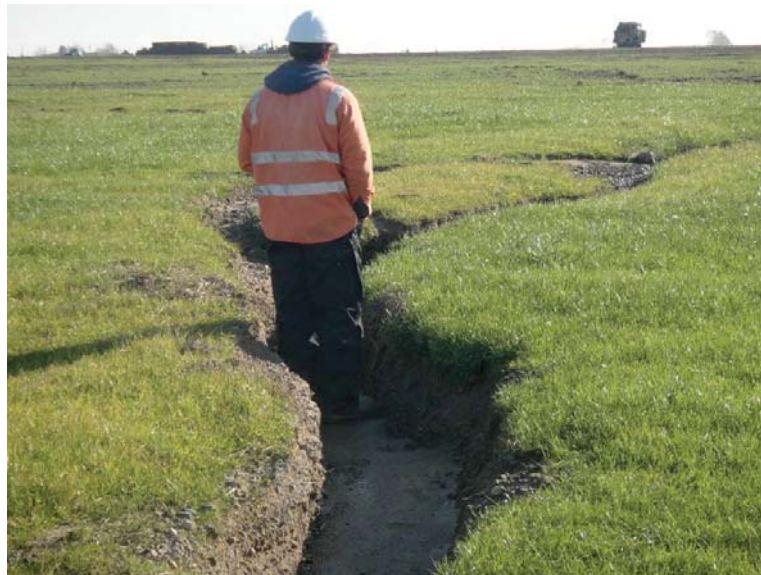
Fig. 5. Seepage erosion feature on the Summit cover system
