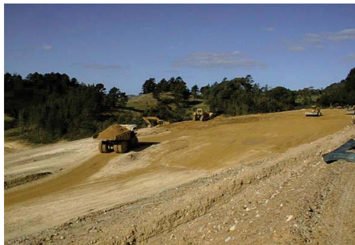
Fig. 5. Construction of encapsulation layers
